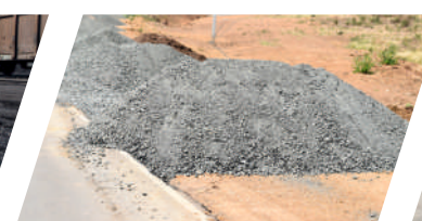
Crusher to Site - Blue Metal
