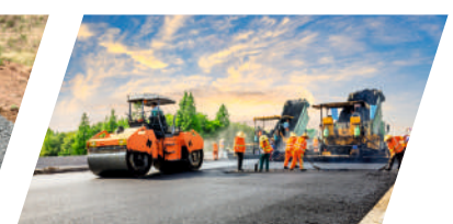
Road Construction Site
